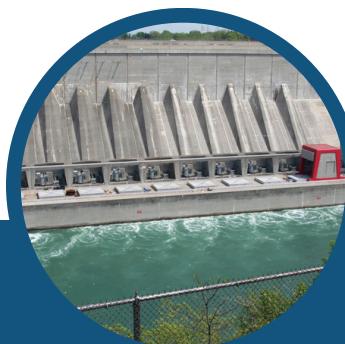
Hydroelectric plant in New York.
