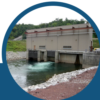
Raystown Hydroelectric Plant.
