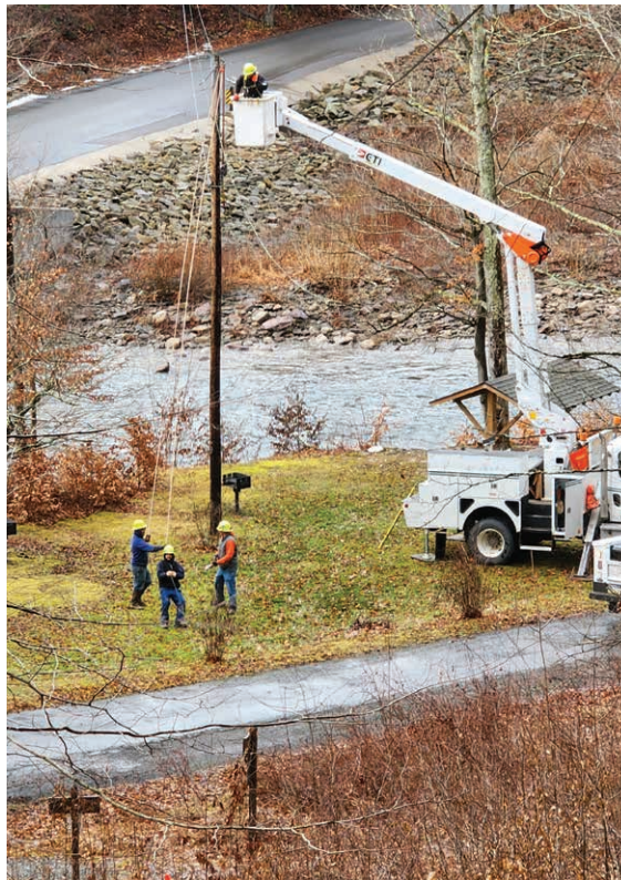
RESTORING POWER: Sullivan County Rural Electric Cooperative lineworkers restore power at Worlds End State Park while climbing poles and working out of a bucket truck. Bucket trucks are a faster alternative to climbing poles, but the terrain lineworkers encounter often prevents trucks from reaching poles and requires crews to climb the poles instead.
