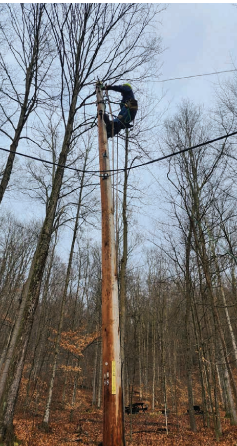
RESTORING POWER: Sullivan County Rural Electric Cooperative lineworkers restore power at Worlds End State Park while climbing poles and working out of a bucket truck. Bucket trucks are a faster alternative to climbing poles, but the terrain lineworkers encounter often prevents trucks from reaching poles and requires crews to climb the poles instead.
