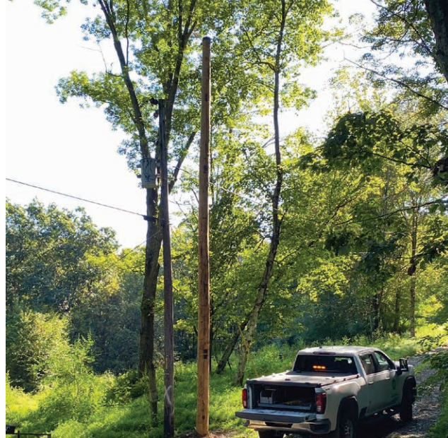
HEIGHT DIFFERENCE: To ensure adequate clearance, communications companies are paying to replace co-op poles so they can safely attach communications lines. This new pole on the right is much taller than the old pole installed in the 1940s.
