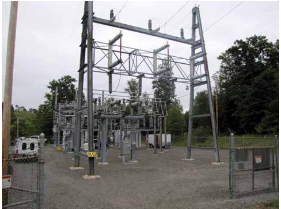
REPAIRS: The Mill Creek Substation is shut down in October so needed repairs could be made. Members normally supplied power from the substation had power backfed to them from other substations while the work was completed.
