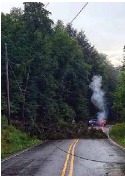
DON'T MOVE: Power lines can come down due to vehicle accidents, trees, snow and ice, etc. If you come across a downed power line, assume it's still energized, and do not attempt to move it. (Laporte Volunteer Fire Company)
