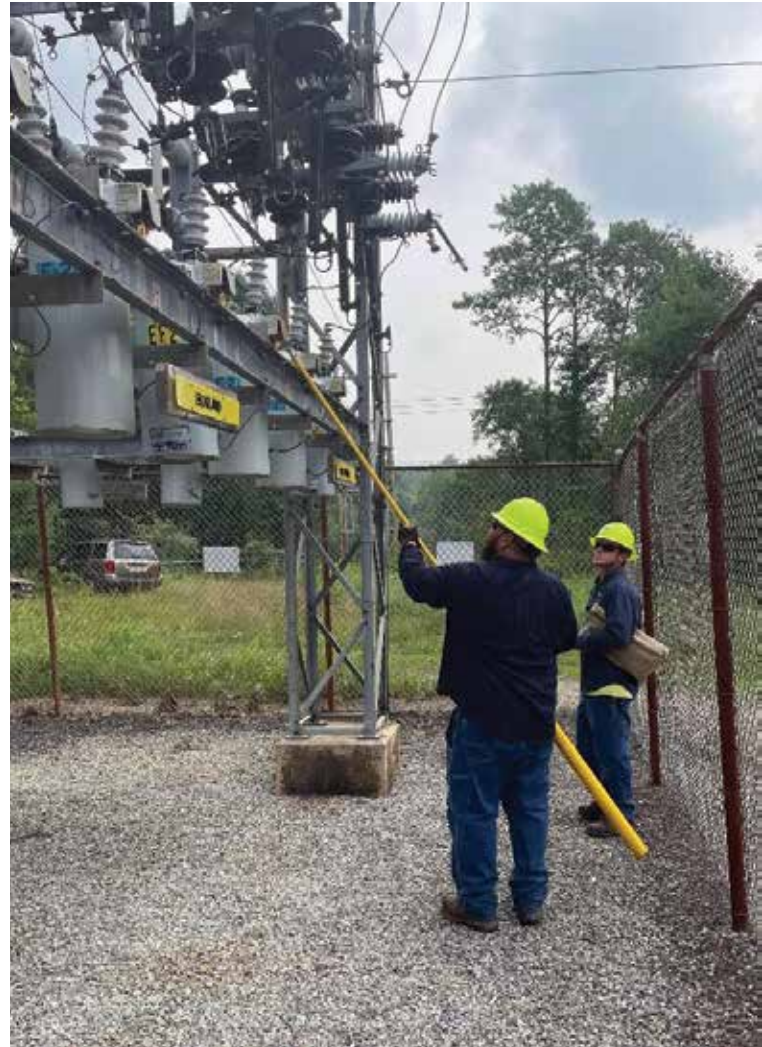
RESTORING POWER: When problems arise, lineworkers can backfeed power to a substation in some situations, but it normally takes around an hour and a half. Here, linemen Tyler Worthen and David Kepner switch power back to the normal feed at the Estella Substation.
