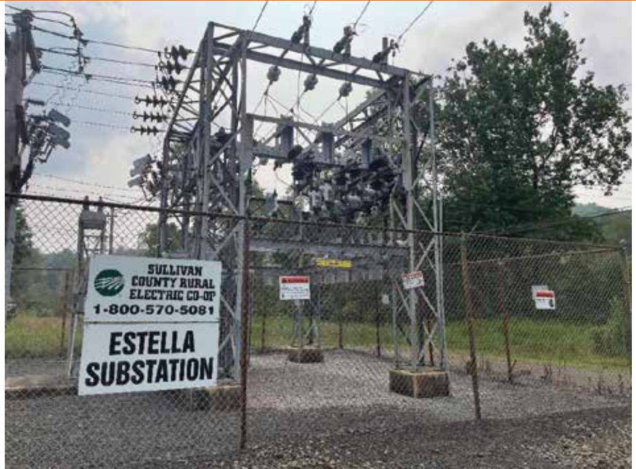
SULLIVAN SUBSTATIONS: Sullivan County REC has five substations. Mill Creek Substation is supplied power by Pennsylvania Power and Light (PPL). Our Estella, Dushore, Kellyburg and Laporte substations are all supplied power by Penelec.
